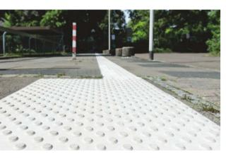
With the aim of enabling blind and visually impaired persons to reach places of information in an unassisted manner, our paste-on DIN 32984 markings alter the floor surface, so that they are easily felt with the cane or the feet or seen due to their increased contrast.
